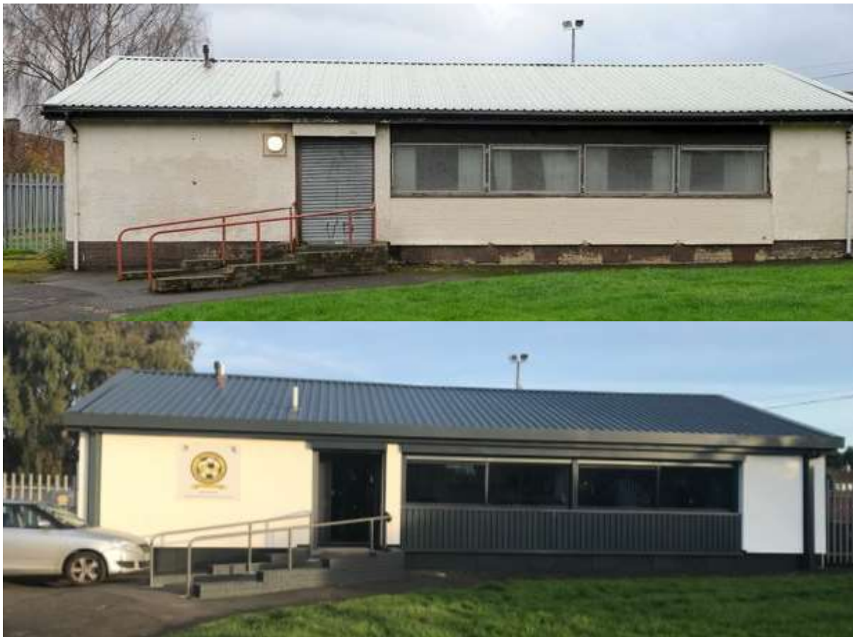
Figure 7 Before and after – external renovations of asset
